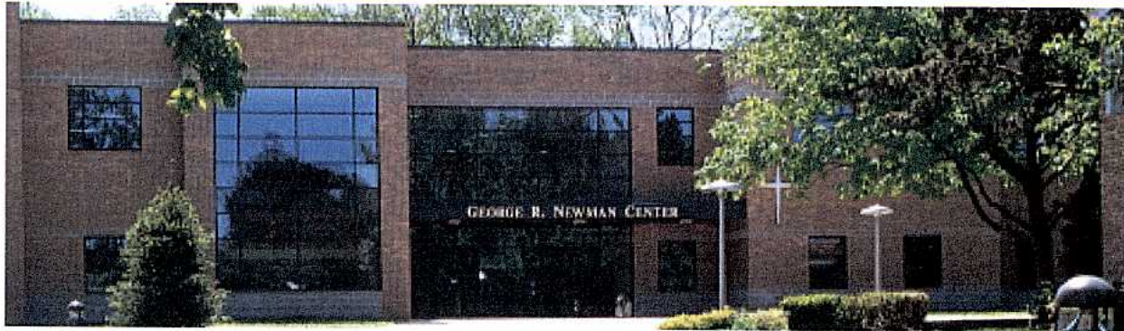
Caldwell College's new $8.5 million George R. Newman Student Activities & Recreation Center
